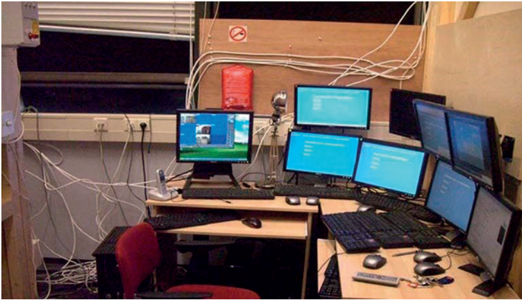
Figure 8. Control room section
